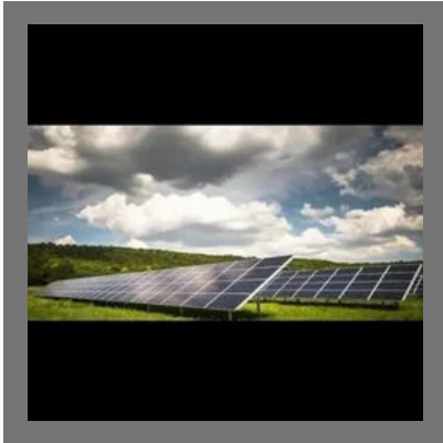
On Grid Solar Power Plant
